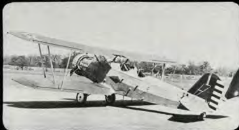
T-2 equipped for blind flying. Right, Maj A. F. Hegenberger, conceived system. First flight 1932, first hooded solo landing on May 9, 1932.
